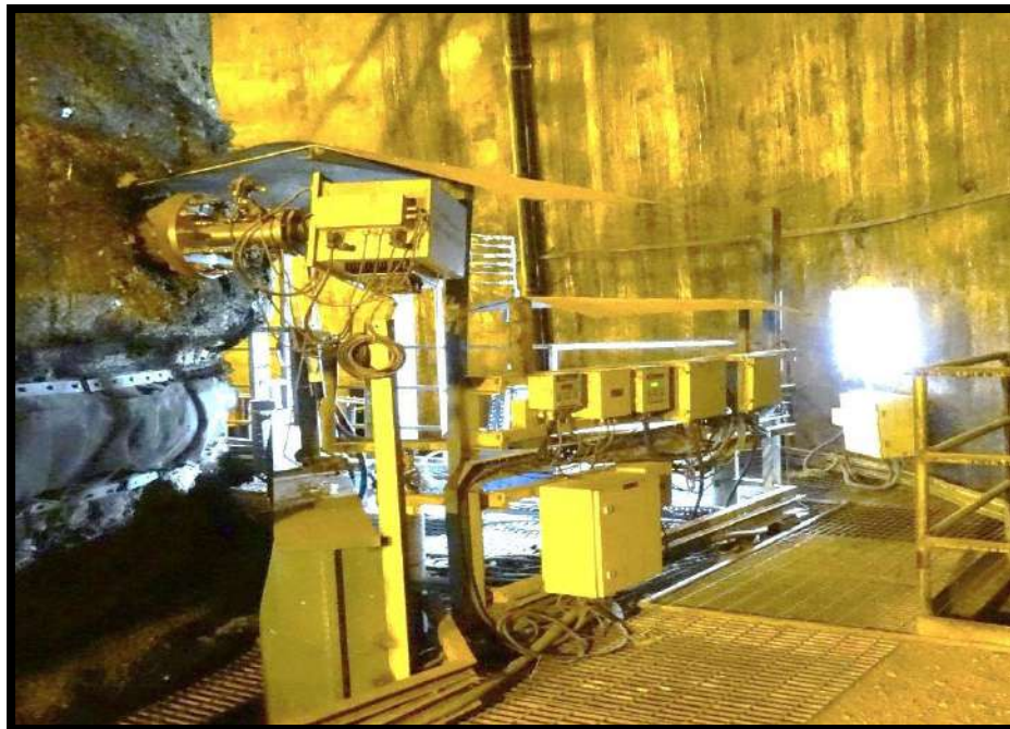
Continuous emission monitoring system installed at main stack for measurement of Particulate Matter & Gaseous Emissions.
